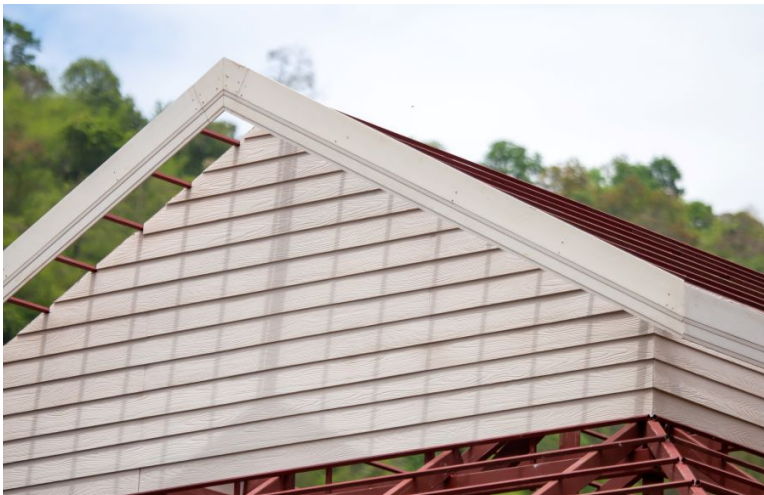
Made with recycled materials, fiber cement siding is more durable and fire-resistant – and less expensive – than wood. But like wood siding, it is not recyclable at end of life.
