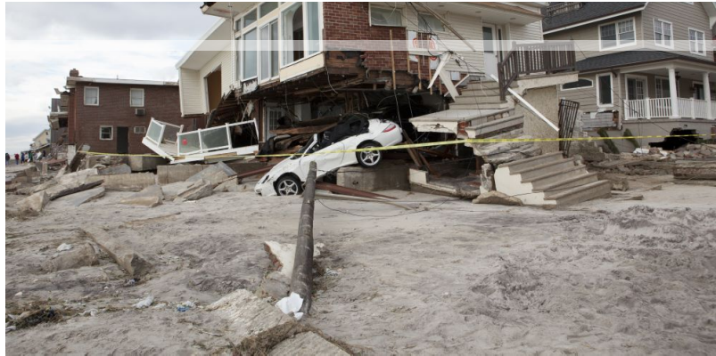
Damaged home after Hurricane Sandy. Source: Adobe Stock
