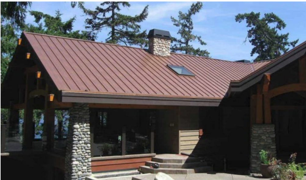
Standing seam metal roofing. Photo: Interlock Lifetime Roofing Systems
